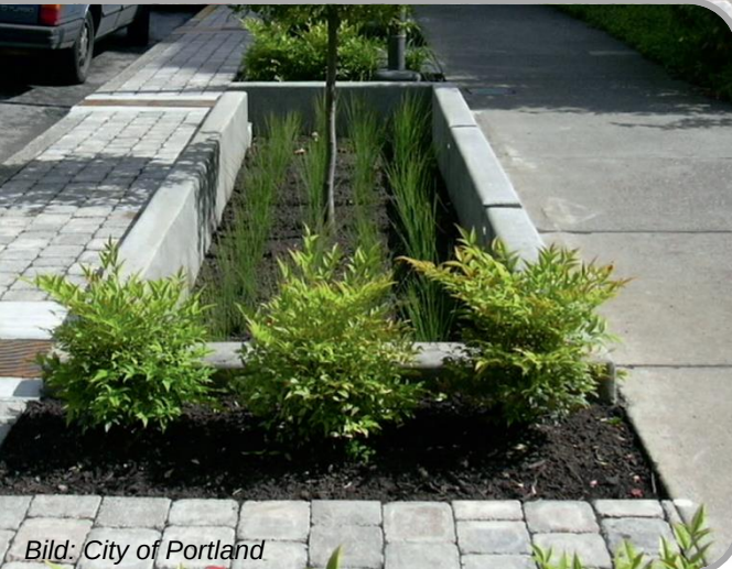
GREEN INLET CARRIES WATER FROM SIDEWALK INTO PLANTER
