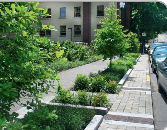
GREEN INLET CARRIES WATER FROM SIDEWALK INTO PLANTER
