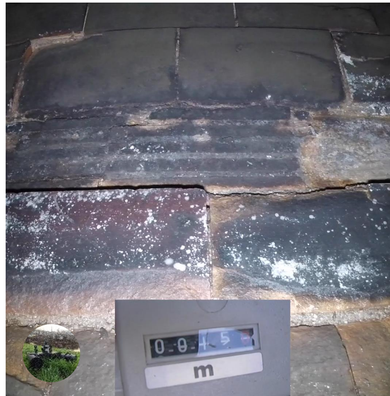
Jena: free-surface pipeline
