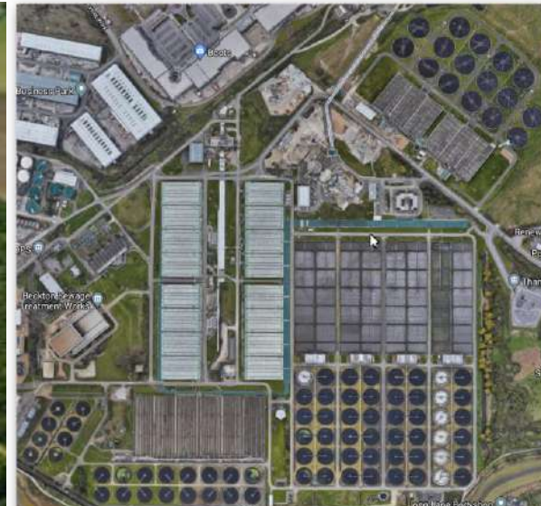
London, Beckton, Thames Water, 3,5 Mio EW, ASP3 N-RTC, SRT-RTC Installation
